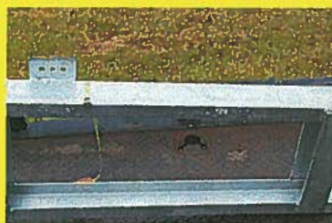
ET-Plus 4-inch guide channel
