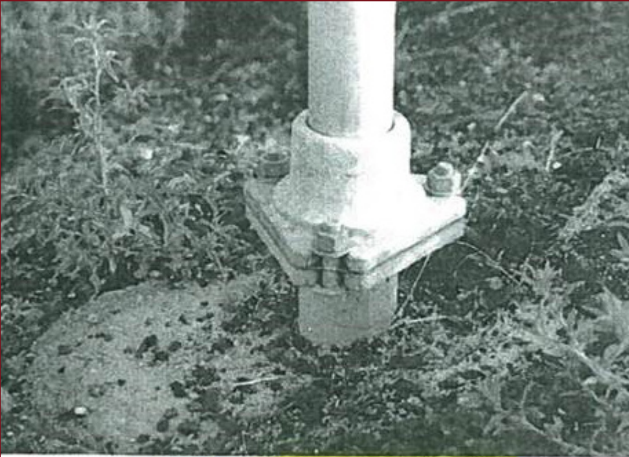
FIGURE 4.9 Multidirectional slip base for small signs
