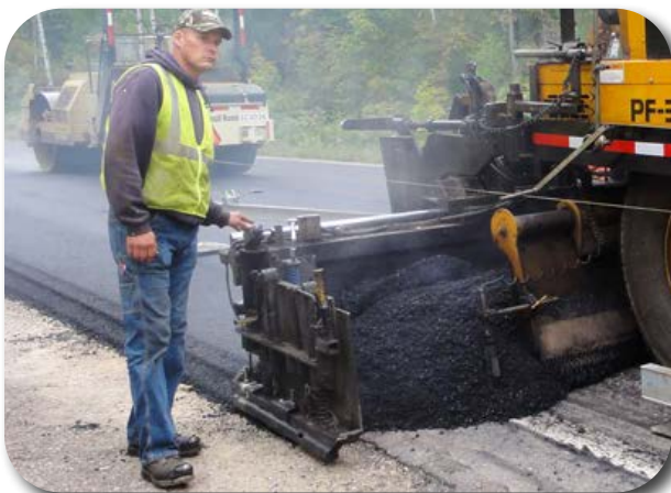
Safety Edge™ installation FHWA website
